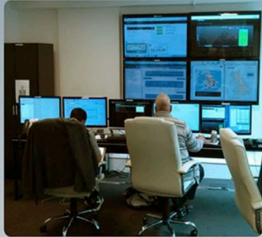
Kiwi Power aggregator interface to National Grid
