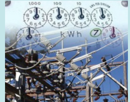
DC and AC Metering (>100kV ac site cal. + dc side meter.)
