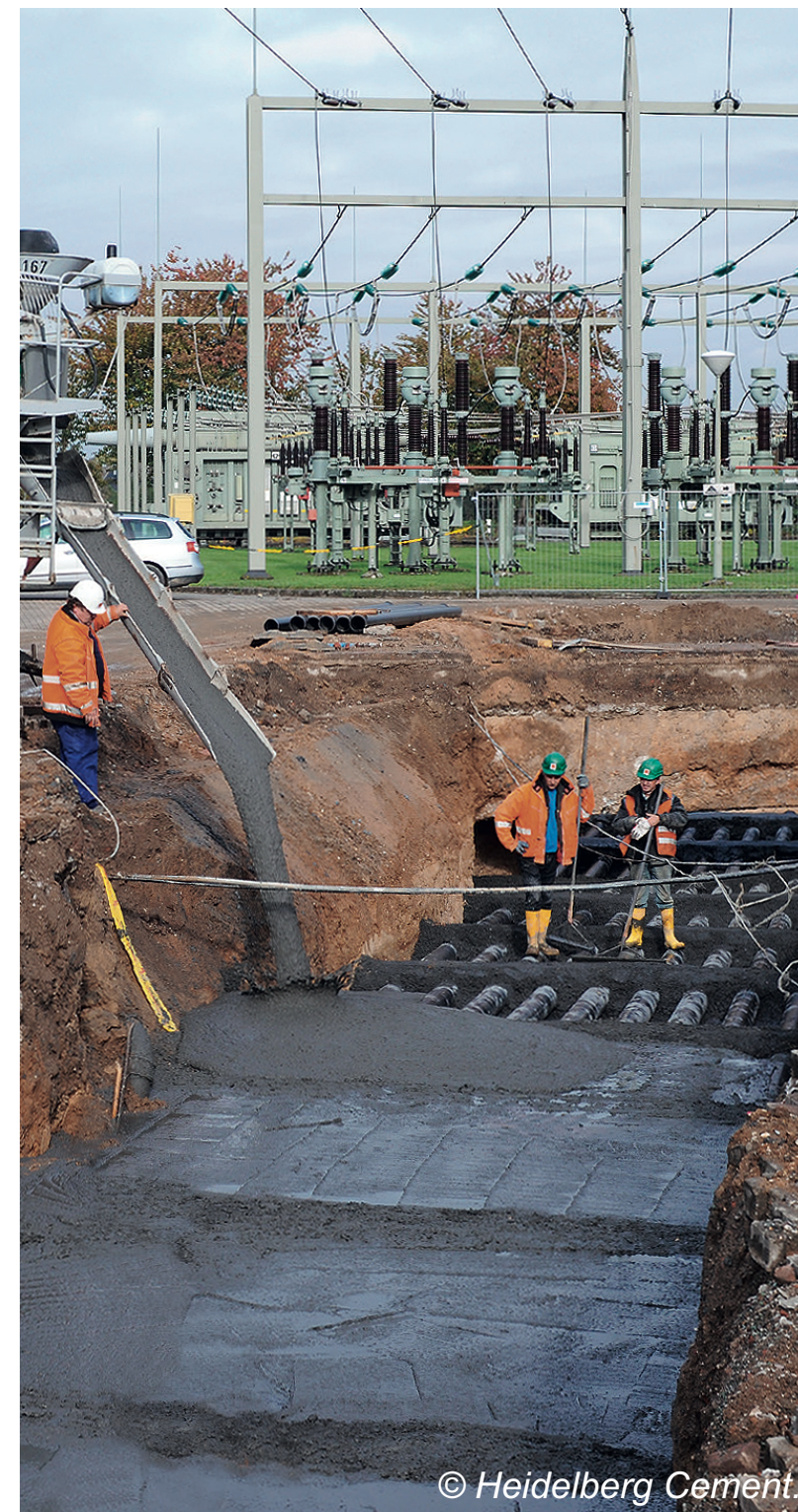
© Heidelberg Cemeht. Thermal concrete in underground power line application.
